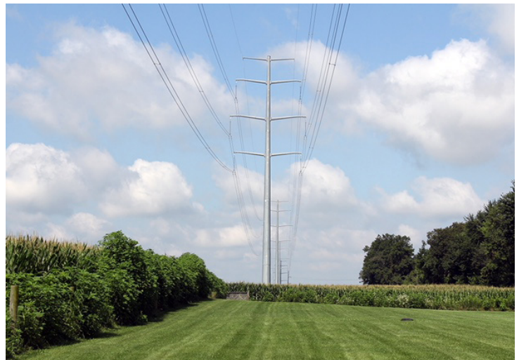
The photograph depicts a typical double-circuit steel monopole. Actual structure type and height may vary along the route. While the structure type may vary, the typical right-of-way is 130 feet wide for safe construction, operation and maintenance of the facilities.
